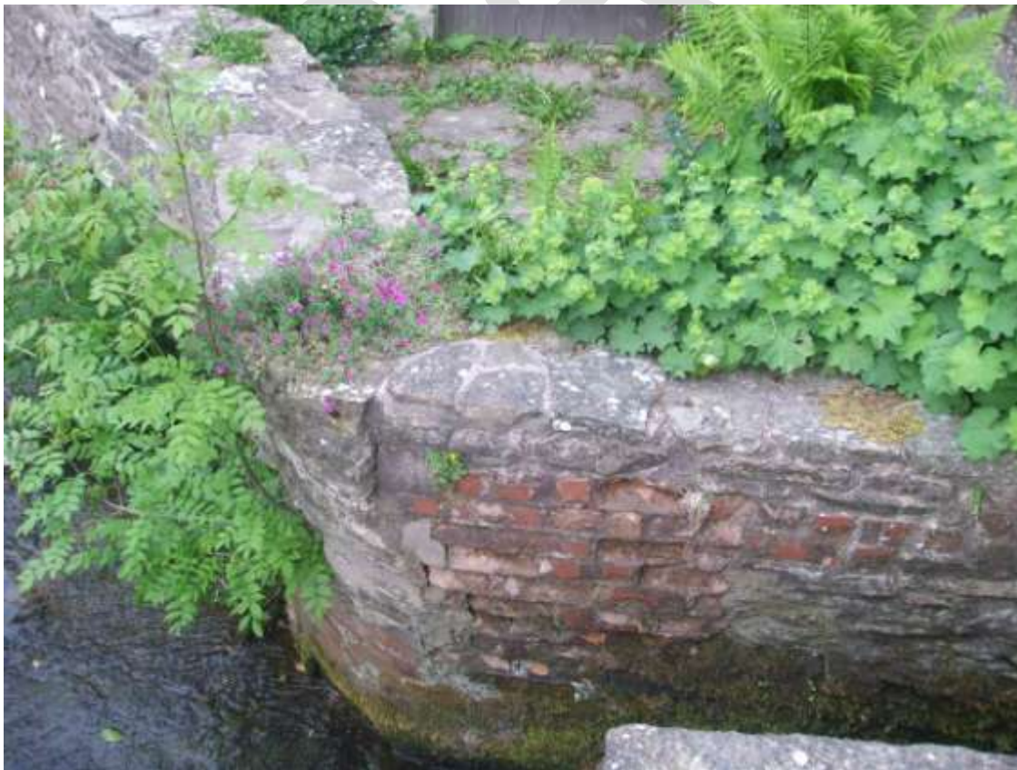
Figure 8: Failing bank wall at corner below mill to be cut back/realigned in concrete
