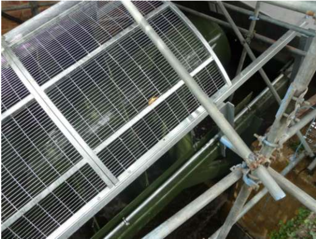
Figure 11: Screw turbine with a mesh cover, during installation
